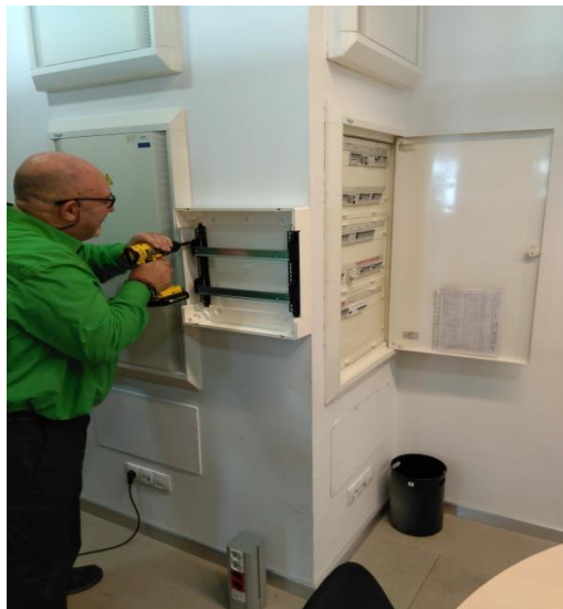
Figure 28: Electrician adding an enclosure to locate the meter outside of the electrical panel compartment
